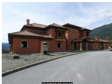
Front facade from upper access road
